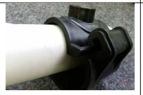
The lower part of the clamp saddle has to be hooked in the upper part of the clamp saddle.
