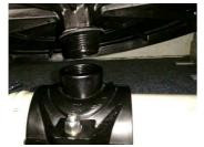
The disc diffuser can be installed now by screwing into the socket of the clamp saddle. Always make sure that the diffuser is firmly and horizontally mounted.
